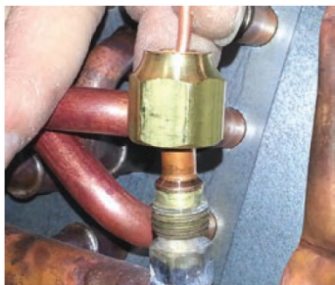
B. Screw flare nut on TXV equalization tube onto the Scradar valve stem.
